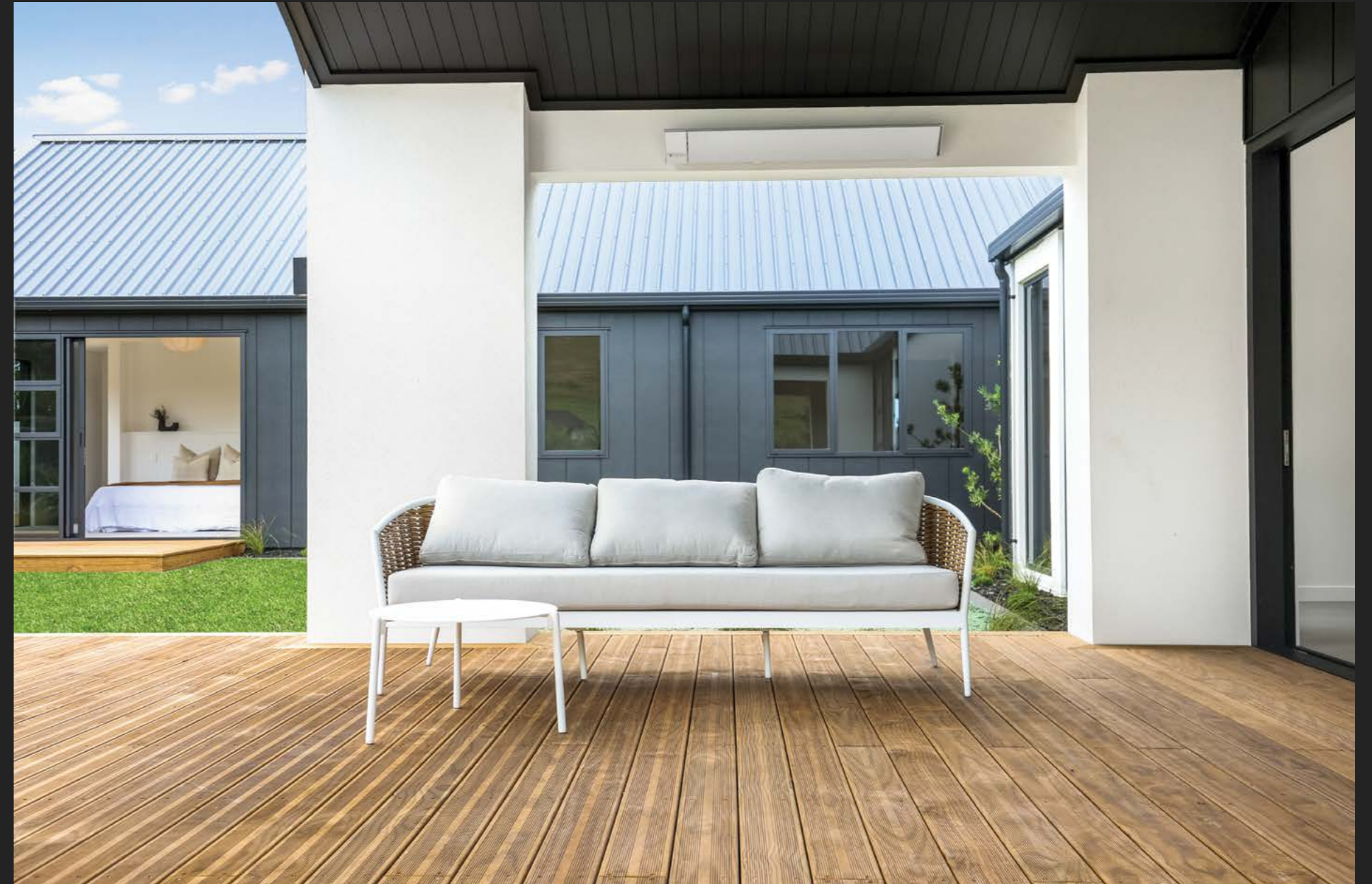
Imbue Radiata Decking, Whatawhata, New Zealand. Installed 2022.
