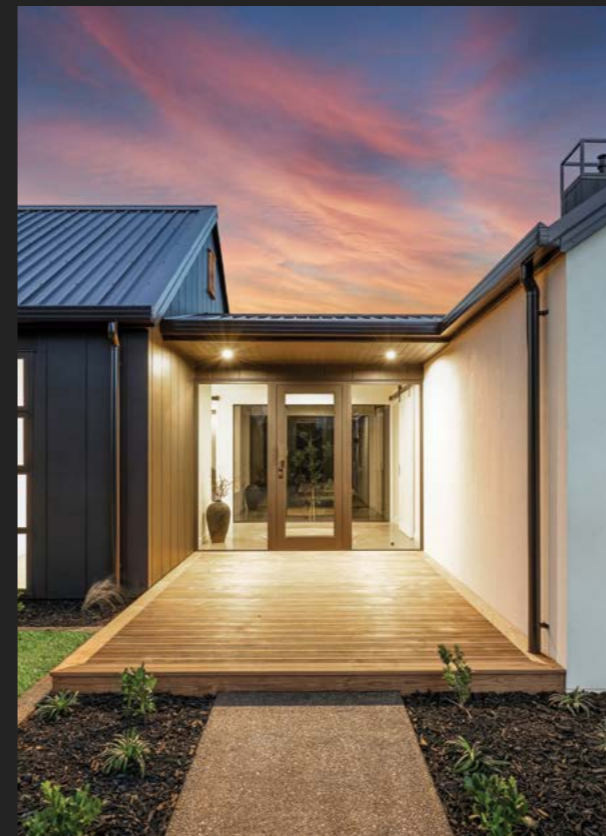
Imbue Decking, Whatawhata, New Zealand. Installed 2022.
