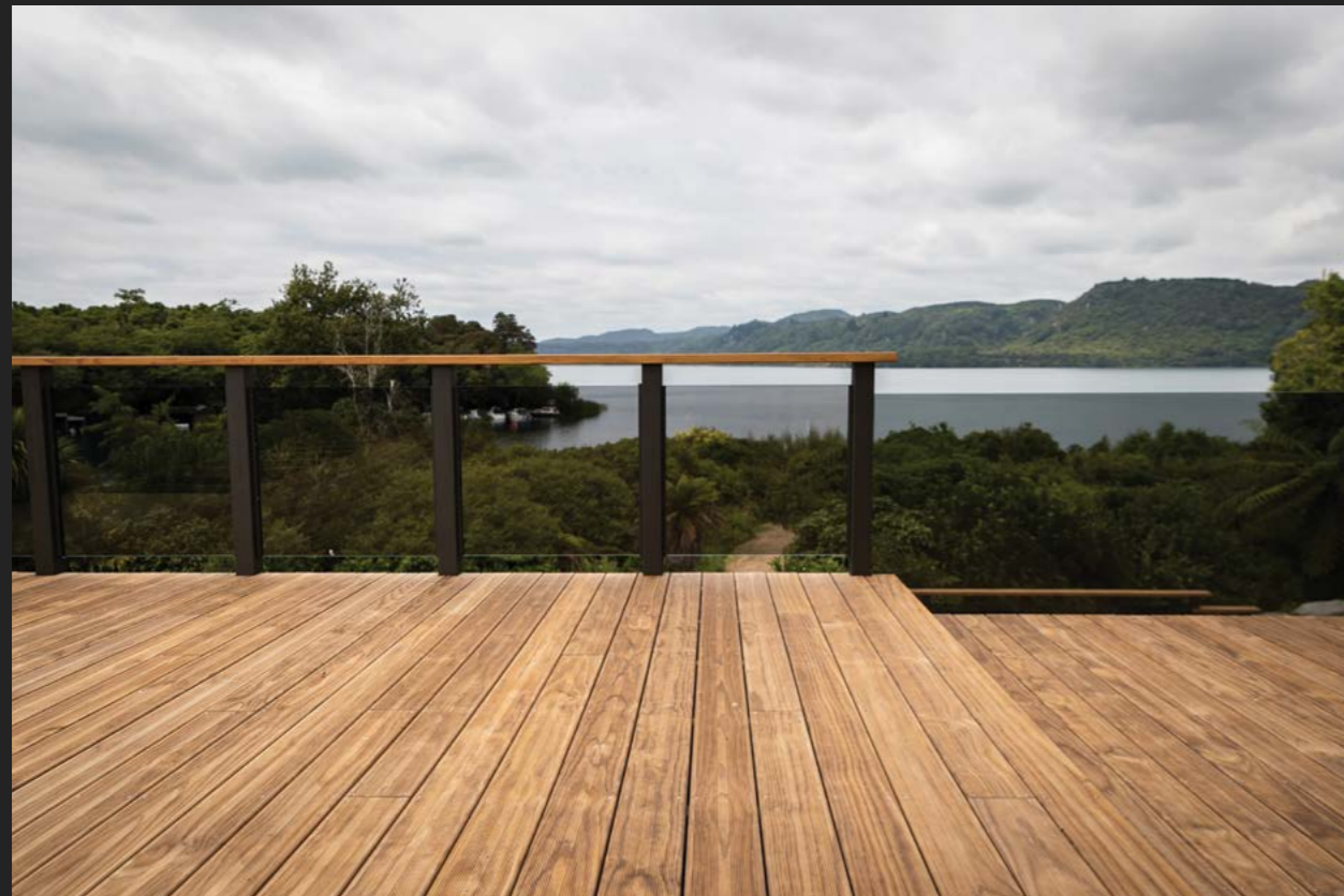
Imbue Decking, Rotorua, New Zealand. Installed 2020.
